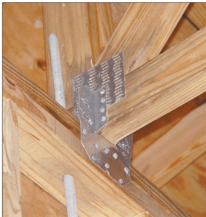
The all thread rods, placed at approximately 60 inches apart around the home, connects from the bottom of the beam to the top plate. The hurricane clip secures the trusses to the top plate developing a continuous hold down system from foundation to top plate.
