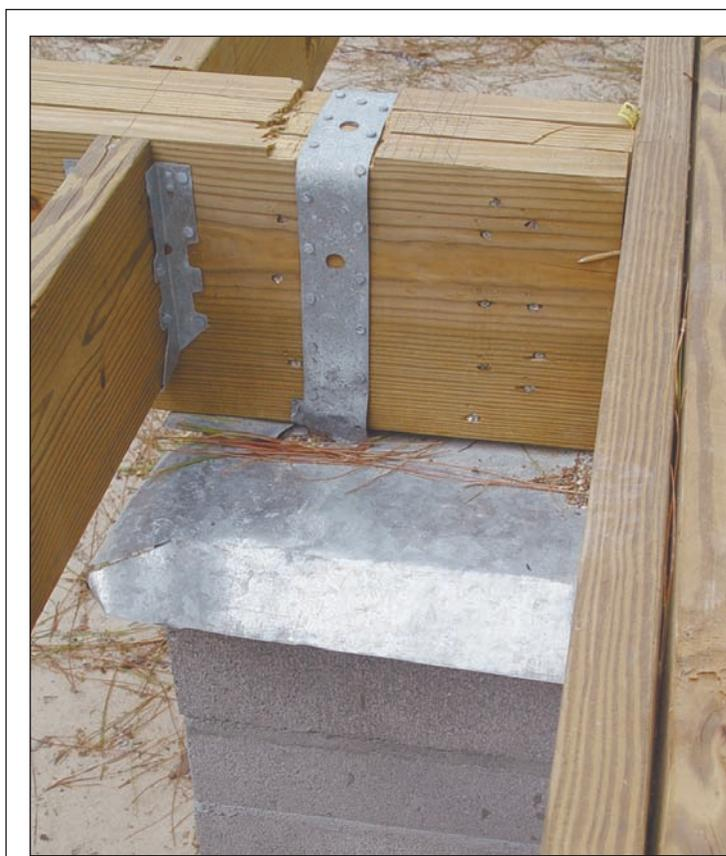
The heavy-duty strap is embedded in concrete and is wrapped around the perimeter beam.
